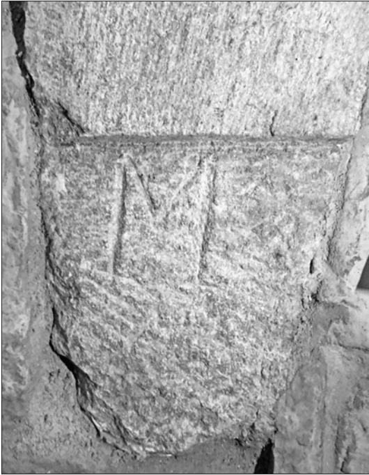
8.3 Stone showing a mason's mark from a wall at Fort de Chartres IV. Perhaps the "M" was incised by Jean Manuel of Prairie du Rocher or Eustache Moreau of Kaskaskia. (Courtesy of Fort de Chartres State Historic Site museum; photograph by the author)
